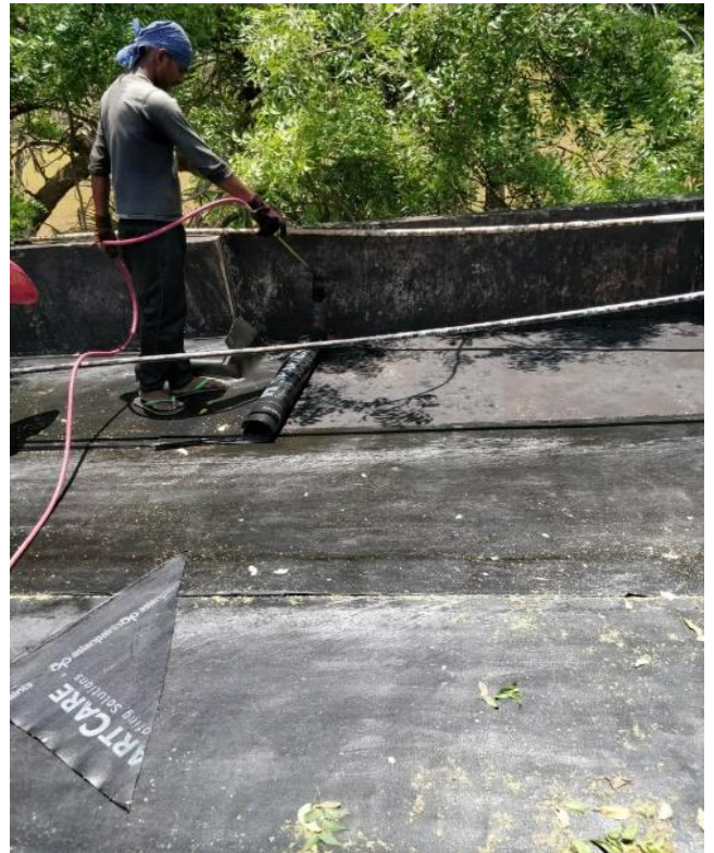
Terrace water proofing with SmartCare APP 3mm Polyester membrane by heat torching method
