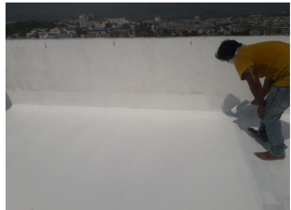
2 nd coat of PU Aqua application; Coating shall be extended to vertical parapet walls of min. 300mm
