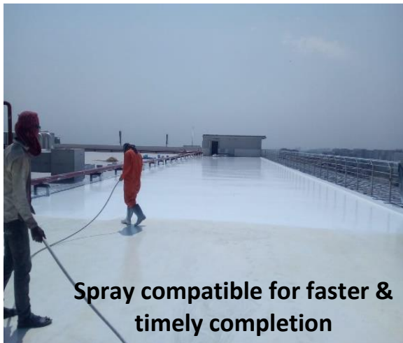
2 nd coat of PU Aqua application; Coating shall be extended to vertical parapet walls of min. 300mm
