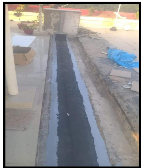
Expansion Joint treatment with SmartCare Hybrid PU sealant
