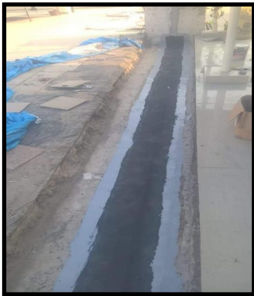
Expansion Joint treatment with SmartCare Hybrid PU sealant
