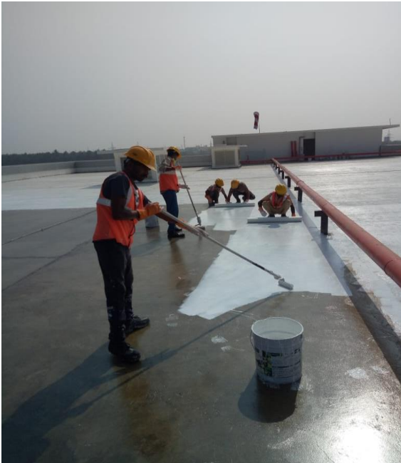
1 st coat of PU Aqua application after clear epoxy primer coating
