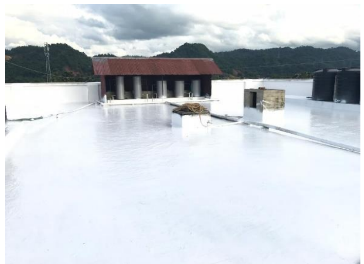
2 nd coat of PU Aqua application; Coating shall be extended to vertical parapet walls of min. 300mm
