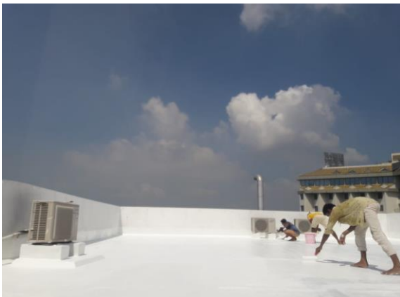
2 nd coat of PU Aqua application; Coating shall be extended to vertical parapet walls of min. 300mm
